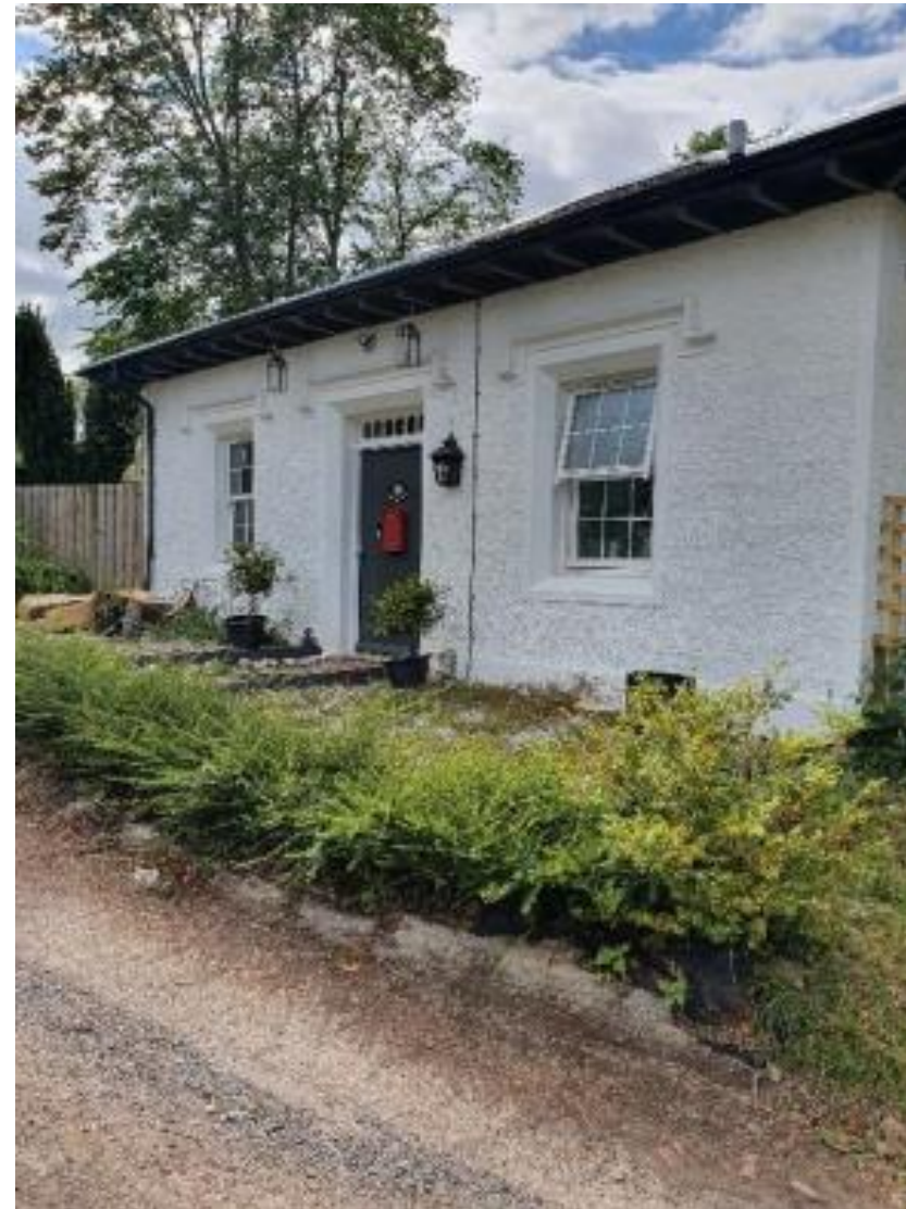
Figure 6: Image of the Existing Cottage
