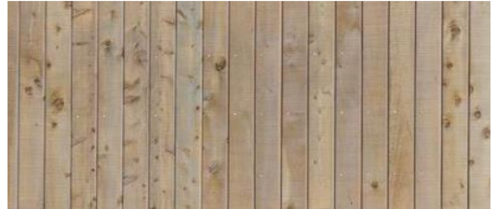
Figure 13: Vertical Timber Cladding
