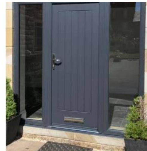
Figure 14: Windows and Doors
